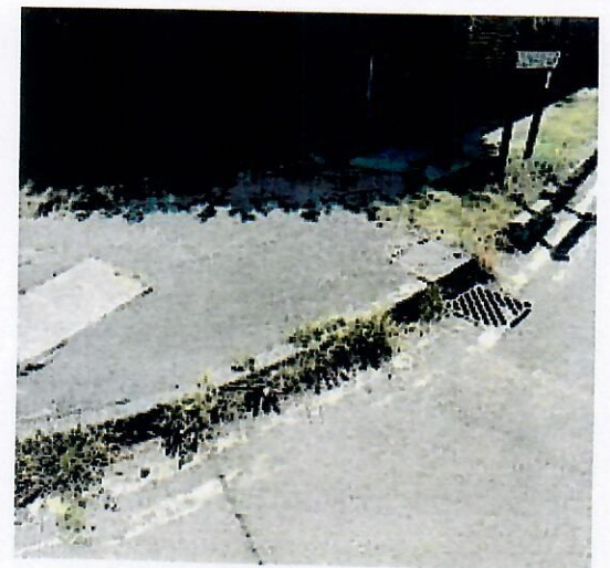
Weeds and vegetation Queensway and Fyfield Road obscuring important road sign warning drivers of a school
